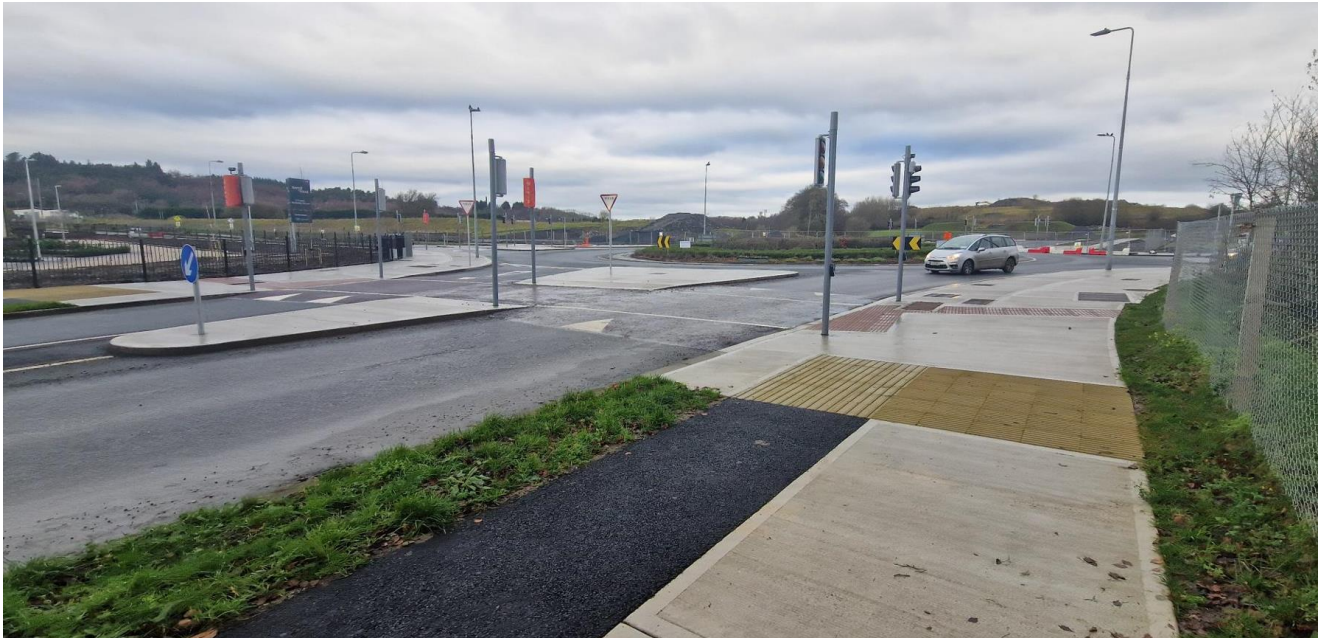
Figure 2: Recently Installed At-Grade Signalised Crossings at Oak Drive Roundabout
